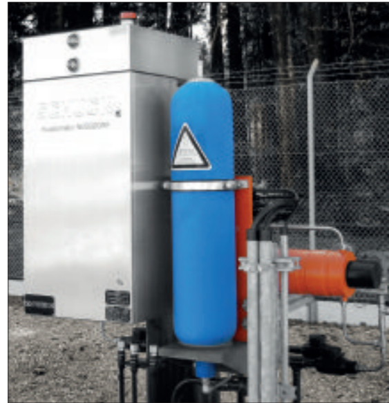
Right: Type C control with remote control OPEN/CLOSE, incl. - Torque limitation - Electronic control Type SEC for monitoring and control of the hydraulic actuator control.
